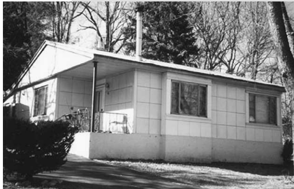
Porcelain enamel finished panels covered the Lustron's exterior. This Lustron found a home in Closter, New Jersey.
