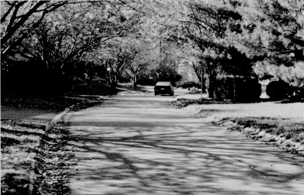
Streets serving only a few homes need only be twenty feet wide
