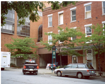
Structured parking can reduce the amount of surface parking lots needed, increasing the overall density that can be achieved in a downtown area. Garages can be designed to blend in unobtrusively, as here in Burlington, Vermont.
