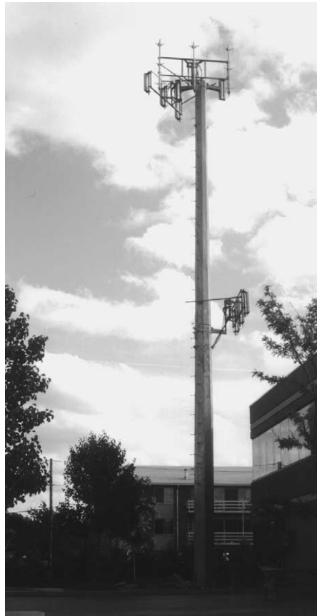
Short monopole ~100' w/split panel array (cellular)
