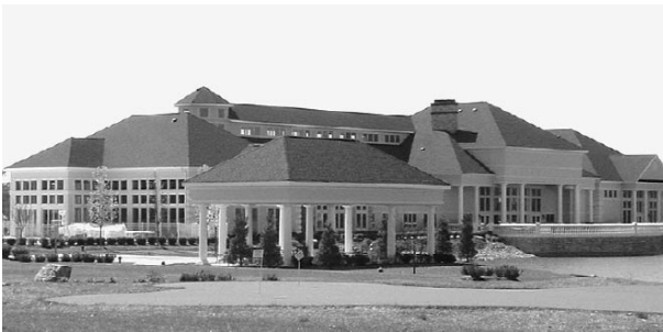
This community facilities building is about 55,000 square feet in size, and includes an indoor pool, a ballroom with a catering kitchen, and many special purpose rooms for exercise, hobbies, and meetings.
