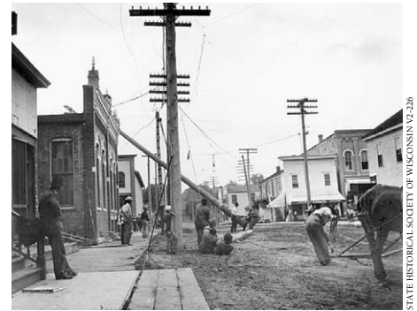
Telephone poles going up in Black River Falls, Wisconsin, circa 1890.
