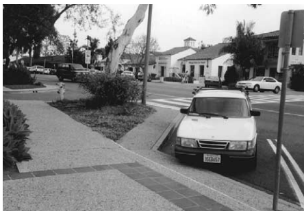
Photo 1. Safe-crosses extend into the street at the intersection so pedestrians are more visible and have a shorter distance to cross. The work with parallel, perpendicular, or angle parking. Note also the bold "Zebra" crossing marks to alert drivers to the crosswalk.
