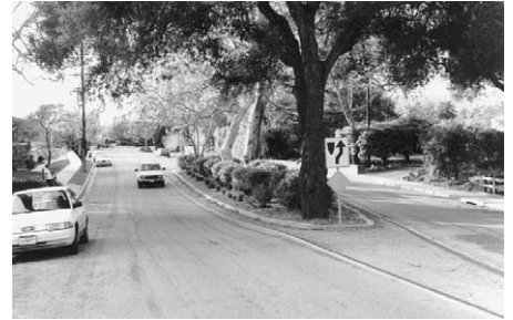
Photo 2. Center islands can be used occasionally to narrow the street and reduce traffic speed.
