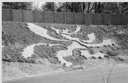
Griffin made of trap rock in a wire mesh casement defines the entry ramp leading from the Blue Route into Radnor Township at Rte. 30
