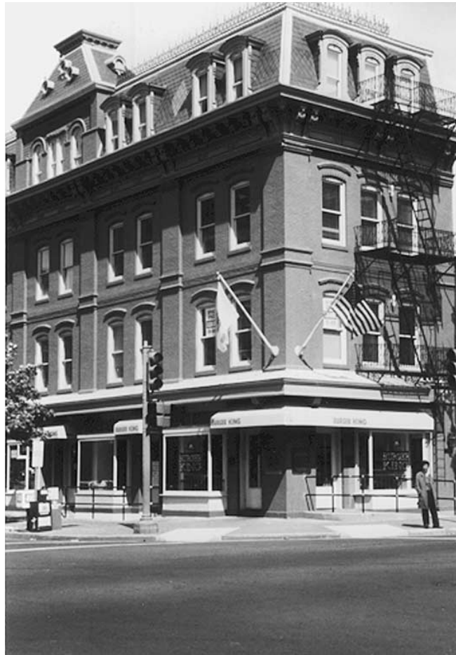
Burger King in restored row structure. Washington, DC.
