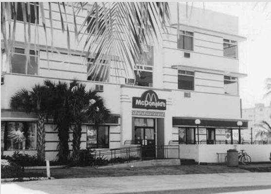
McDonalds in existing building. Ft. Lauderdale, FL
